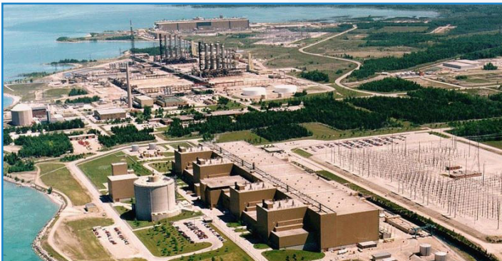
Bruce Power Nuclear Station
